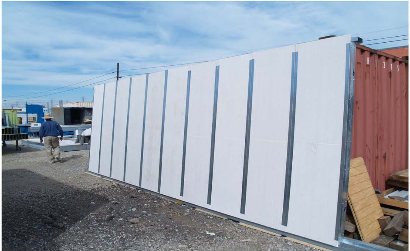
2' X 8' WALL PANELS FOR CHS THERMAL SHEATHING HOME
