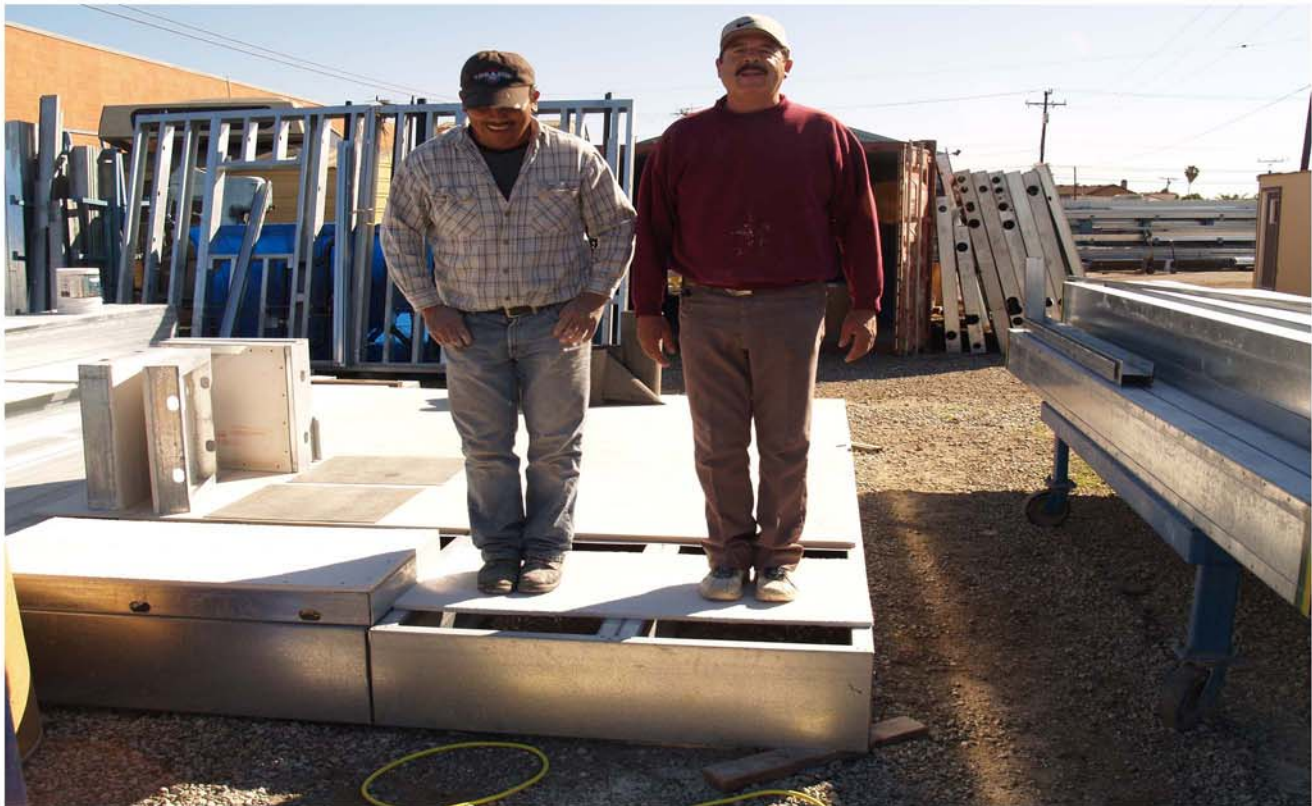
TWO WORKERS (220 LBS & 210 LBS) STANDING ON 24" X 24" SQUARE SHEATHING MAT'LS. FOR LOAD TEST
